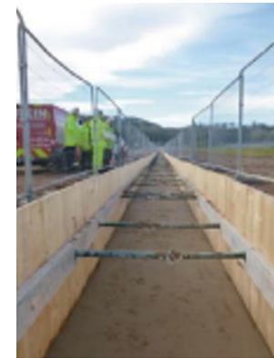
Cable joint bay on a directly buried cable
