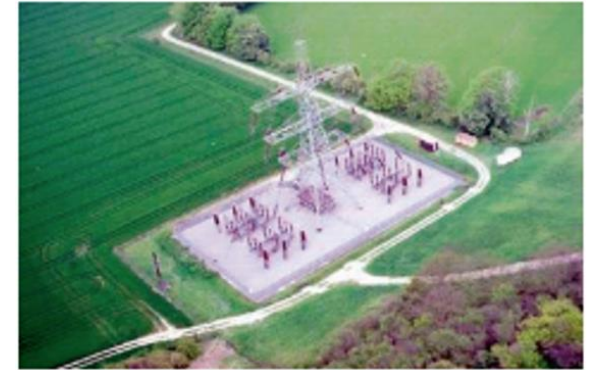
A typical sealing end compound for a directly buried cable
