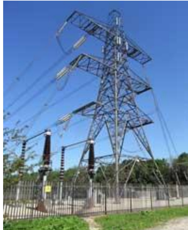
Sealing End Compound in Oxford
