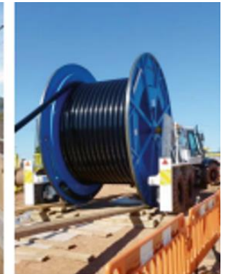
Cable drum offloading cable on site
